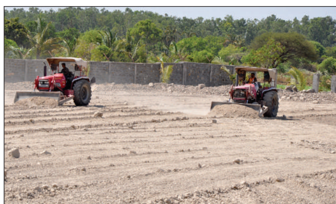
Step 6: Levelling of field plots
