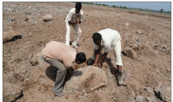
Step 3: Removal and collection of the heavy boulder for road filling
