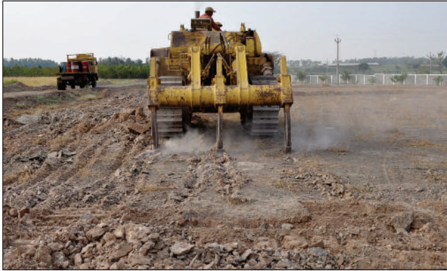
Step 1 : Ripping/chaining of rocky surface
