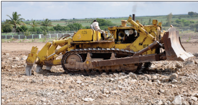
Step 1 : Ripping/chaining of rocky surface
