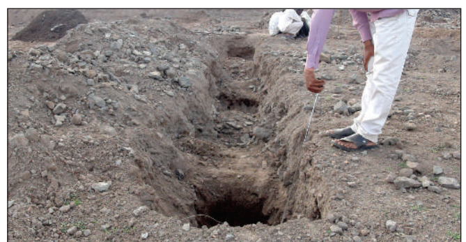
Pits after blasting below plantng sites
